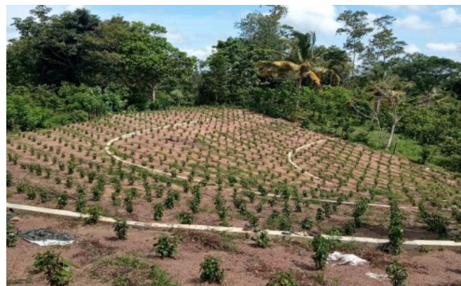
Figure 2 Established concrete bends along the contour line to control soil erosion
