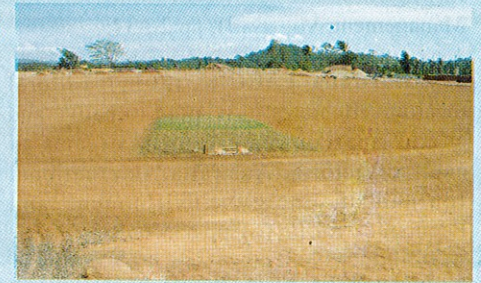
University playground in progress
