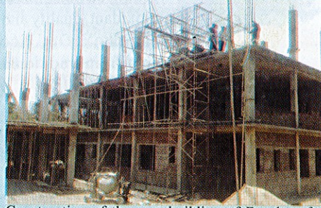
Construction of the new building of Faculty of Geomatics
