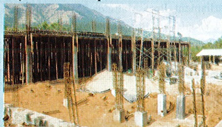
New hostel complex being constructed
